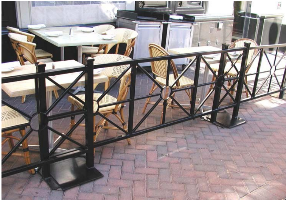
Acceptable sectional fencing design: freestanding
