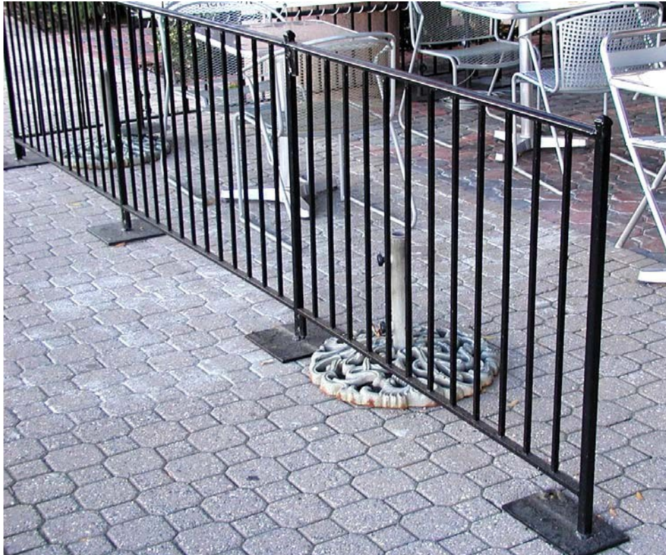
Acceptable sectional fencing design
