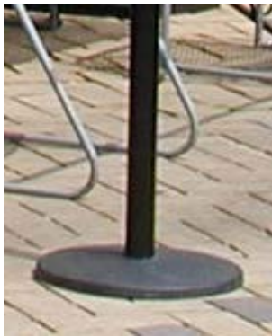
Stanchion base must be flat and no more than 1 1/2" above sidewalk surface
